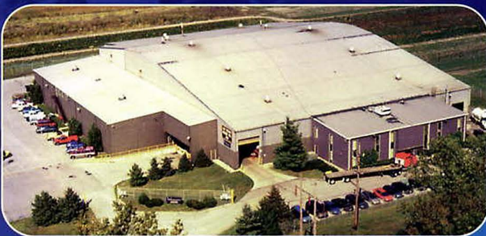
State of the Art 100,000 Sq. Ft. Facility
